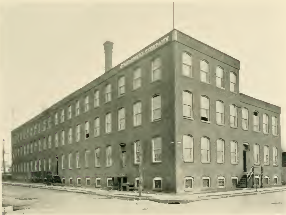
J. RUMMELL COMPANY, PENNINGTON COR., DAWSON STREET.
